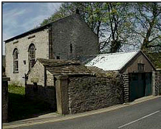
Exterior view of the TSG Chapel Works
